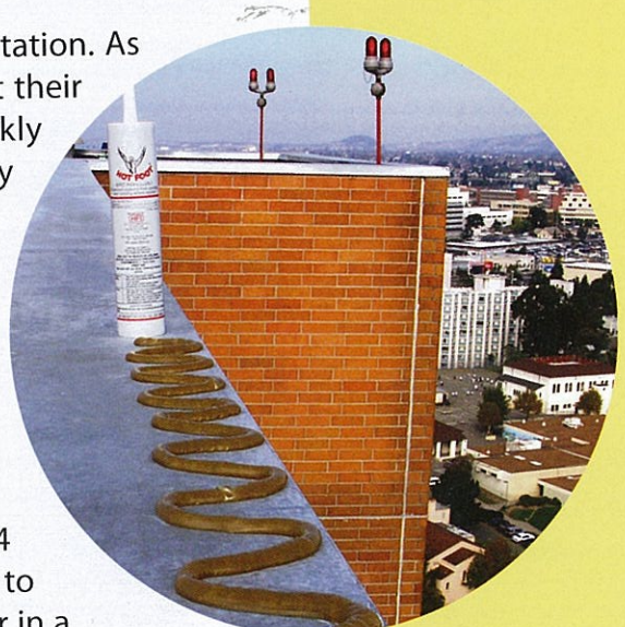
Hot Foot Gel properly applied along a parapet wall.
